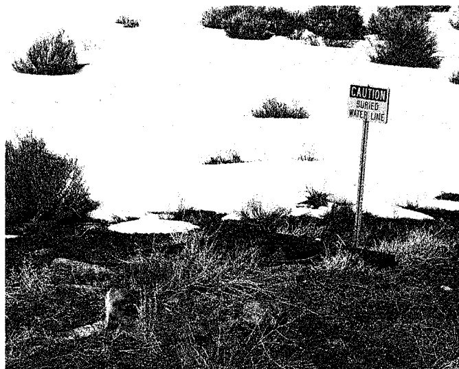
D: Sign states Waterline w/ Manihole- below Human Resource bldg. Waste goes here to natural wash.
