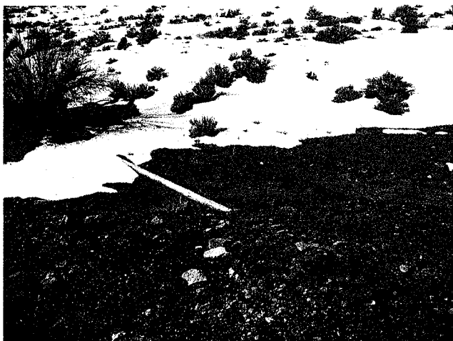
E: waste line exposed to dump in natural wash
